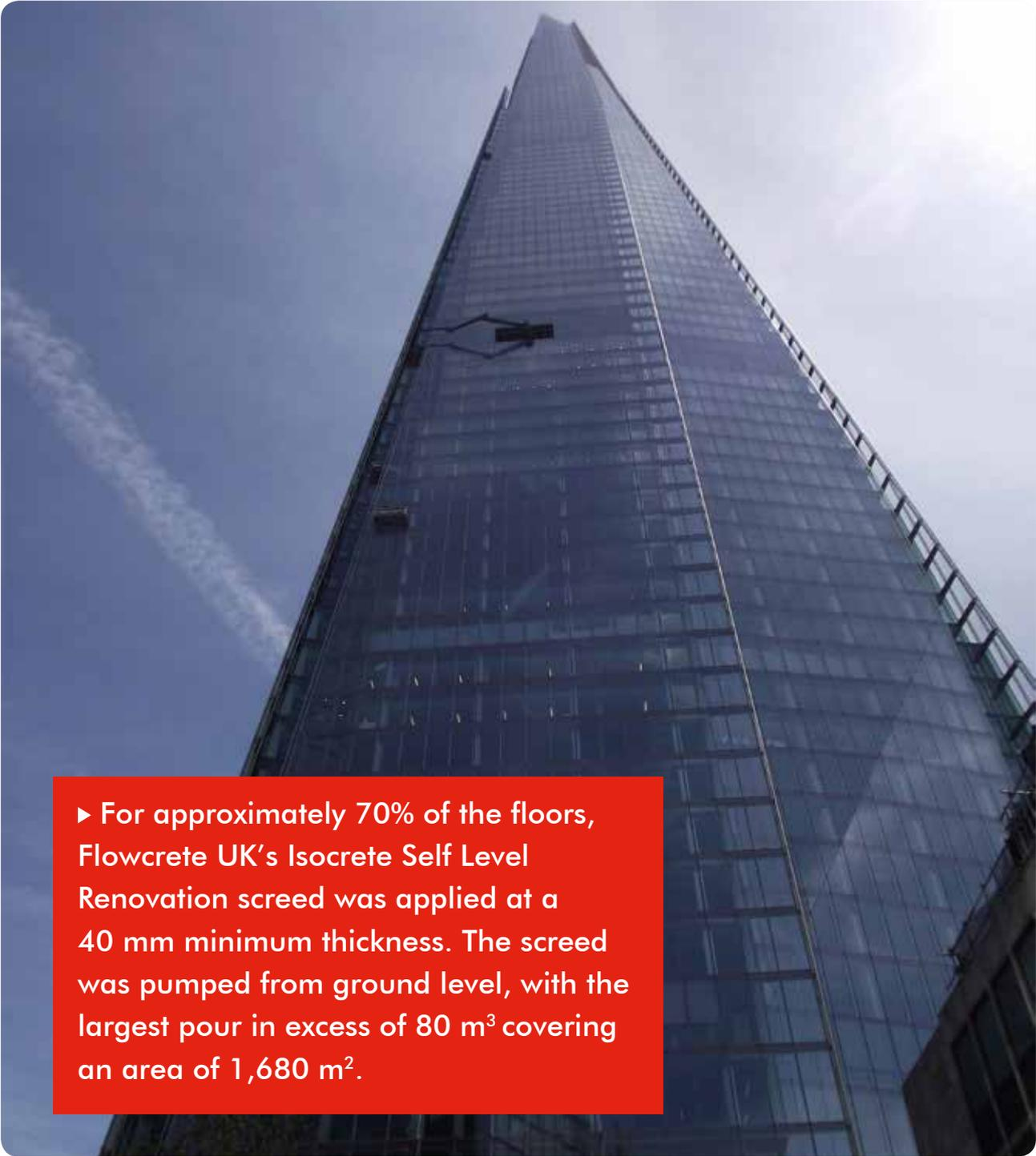
► For approximately 70% of the floors, Flowcrete UK's Isocrete Self Level Renovation screed was applied at a 40 mm minimum thickness. The screed was pumped from ground level, with the largest pour in excess of 80 m<sup>3</sup> covering an area of 1,680 m<sup>2</sup>.
