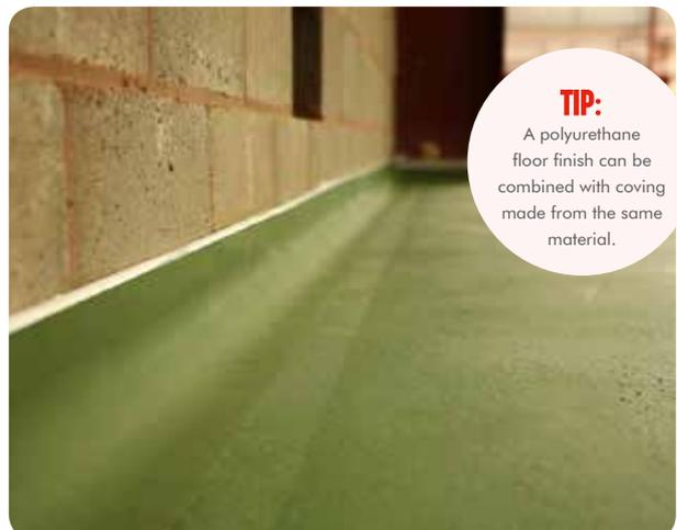
install an expansion joint between the floor and coving. Both products are also independently rebated into the concrete.
