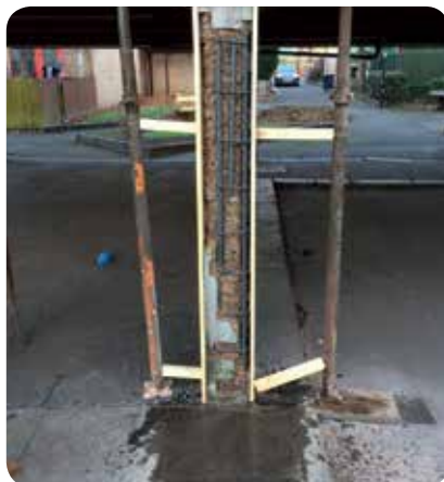
Vertical & Overhead Repair
