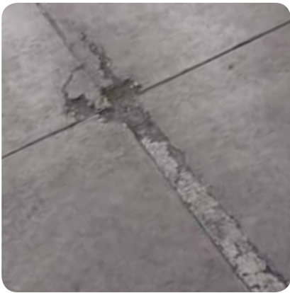
Spalling Joints
